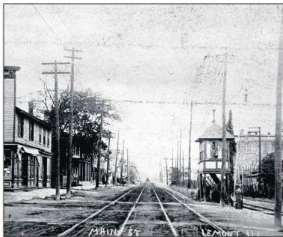
Railroad tracks run through downtown Lemont in 1913. A recent blog post tells of events from 116 years ago that are similar to today's pandemic.
